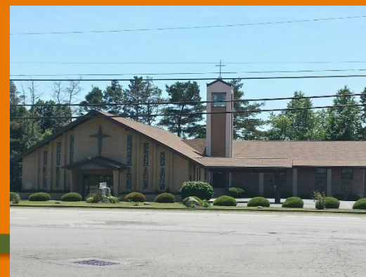
The outside of Valley Baptist Church.
